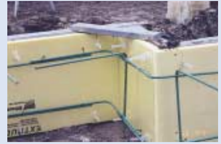
Cox Development, Norfolk, Nebraska, uses plywood forms for monolithic slabs. Plastic ties are preinstalled to fasten insulation to the slab, and steel rebar, to strengthen the slab edge. House on the left is built on a shallow FPSF, except that the foundation of the unheated garage on the right extends to the frost line.
