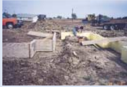
Cox Development, Norfolk, Nebraska, uses plywood forms for monolithic slabs. Plastic ties are preinstalled to fasten insulation to the slab, and steel rebar, to strengthen the slab edge. House on the left is built on a shallow FPSF, except that the foundation of the unheated garage on the right extends to the frost line.
