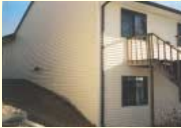
Left, home built by Bill Eich in 1990 in Spirit Lake, Iowa. Garage on the left, built on a FPSF, is attached to a walkout basement with a FPSF at grade (three foundation depths). Siding is straight. No differential movement has occurred.
