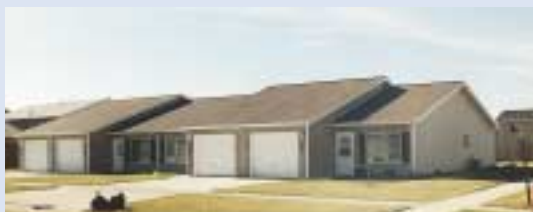
Housing for the elderly and disabled. Eid-Co Buildings, Inc. Fargo, ND. Living space is on shallow monolithic slabs, while garages are on permanent wood foundations. One extends to the frost line while other garages have FPSFs designed for unheated buildings.
