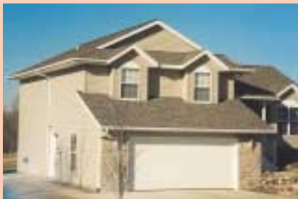
Split-foyer home built in 1996 by Bill Eich, Spirit Lake, Iowa. Right side is a full basement (a conventional deep foundation) while the left side garage and walk-out basement are on frost-protected shallow foundations.
