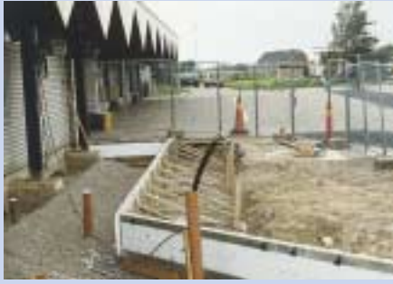
Left: Airport terminal addition at Angelholm, Sweden, using EPS-concrete stay-in-place forms (Skanska Construction)
